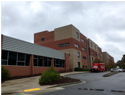
8). Southern Exterior Elevation - Jan 25, 2020
