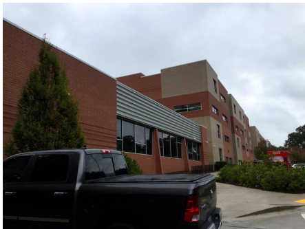
7). Southern Exterior Elevation - Jan 25, 2020
