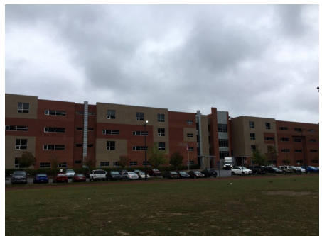
9). Southern Exterior Elevation - Jan 25, 2020
