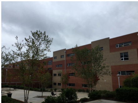
10). Southern Exterior Elevation - Jan 25, 2020
